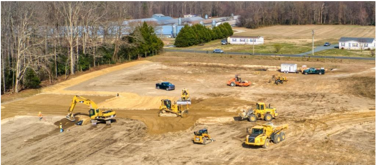
Entry Garden under construction
